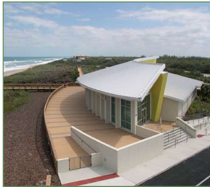
The Barrier Island Management and Education Center
